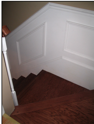
Tight 90 degree turn with limited headroom.
